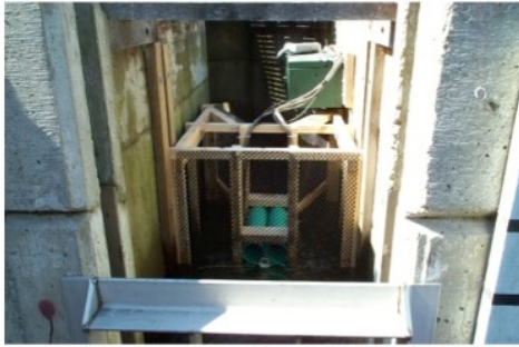
Electronic fish counter and weir at the exit of the Mary Steube Fishway.
